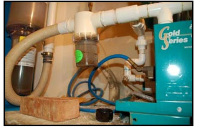
In order to qualify for the Ohio Good DEED program, an ISO 11143 compliant amalgam separator like the Solmetex pictured above must be in use in dental offices that place or remove amalgam.
